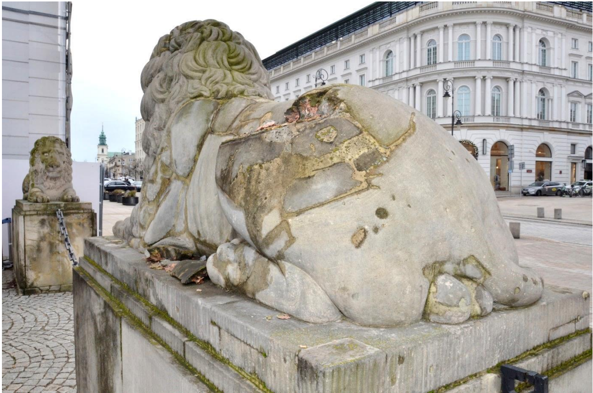
Wojciech Roman, Lion L3 – rump view . Note the completely detached stone fragments (stacked next to the sculpture), [in:] Program prac konserwatorskich [The conservation work programme] , developed by Wojciech Roman, Warsaw 2023, photo 38, page 41.
